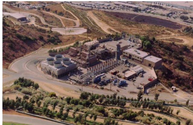
Figure 3 - The Los Angeles County Sanitation District (LACSD) in California has operated a 50 megawatt (MW) landfill gas energy project at its Puente Hills Landfill since 1985, producing electricity for customers throughout Los Angeles.
