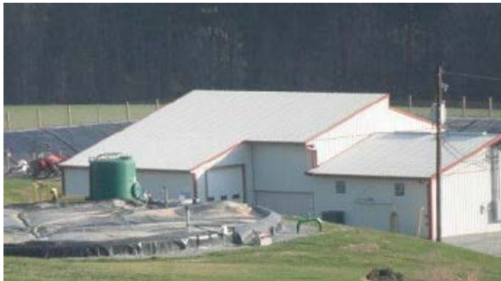
The community digester at Sensenig Dairy in Kirkwood, Pennsylvania is fed six times a day with manure from cows, hogs and chickens, and community food waste. The project has reduced emissions and operational costs, while creating additional revenue from the sale of carbon credits, fertilizer, and bedding.
